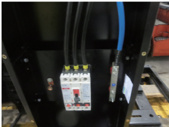
UL/CSA Approved Main Line Circuit Breaker
